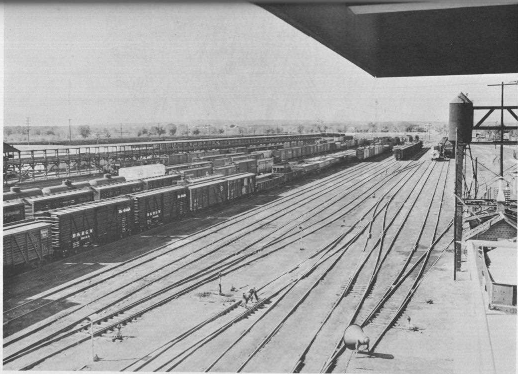
JOINT TERMINAL AND INTERCHANGE YARD (D.&R.G.W.—M.P.), PUEBLO, COLORADO
